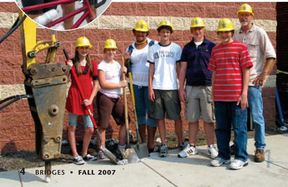
Top photo at left: Janet and John Weber. Bottom photo: A Kraybill class studying construction is using the Kraybill Campus renovations as a hands-on case study in project planning and implementation. Using actual Kraybill project documents, the class learned about the planning that goes into construction, including permits, zoning, site plans, environmental issues, and storm water run off. The class plans to assist with some demolition work and observe and discuss the construction. The students also may do some interior painting of the Kristin Palazzo Gallery. Class members included here with shop/home technology teacher James Baer (far right) are, left to right: Becca Slack, Chelsea Book, Alleayah Myers, Alex Nissley, Lucas Meador and Steven Travis.
