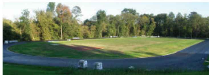
The new track and field facility, to be completed by the end of October, features a rubberized surface.
