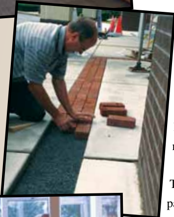
Right: Jim Baer installs bricks along the new pathway to the entrance.
